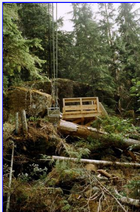
The "new" cable car crossing at the 11 km mark over the drinkwater creek [Ken Rodonets photo]
