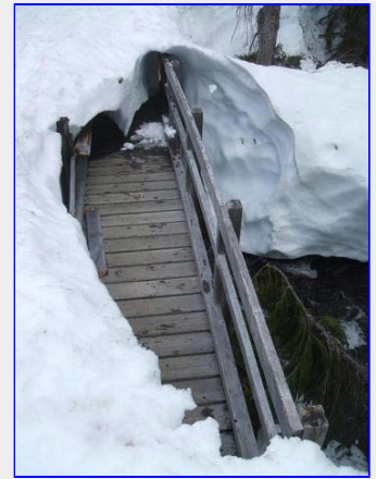
Piggott Creek bridge [Bob St.John photo]
